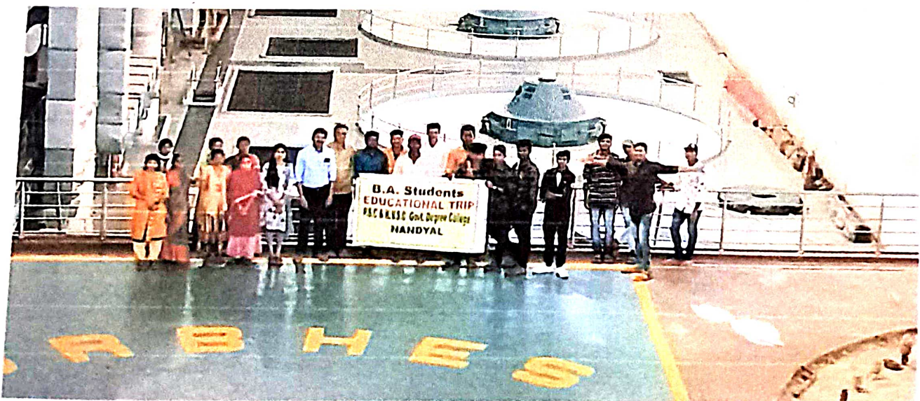
INSIDE OF THE POWER HOUSE
